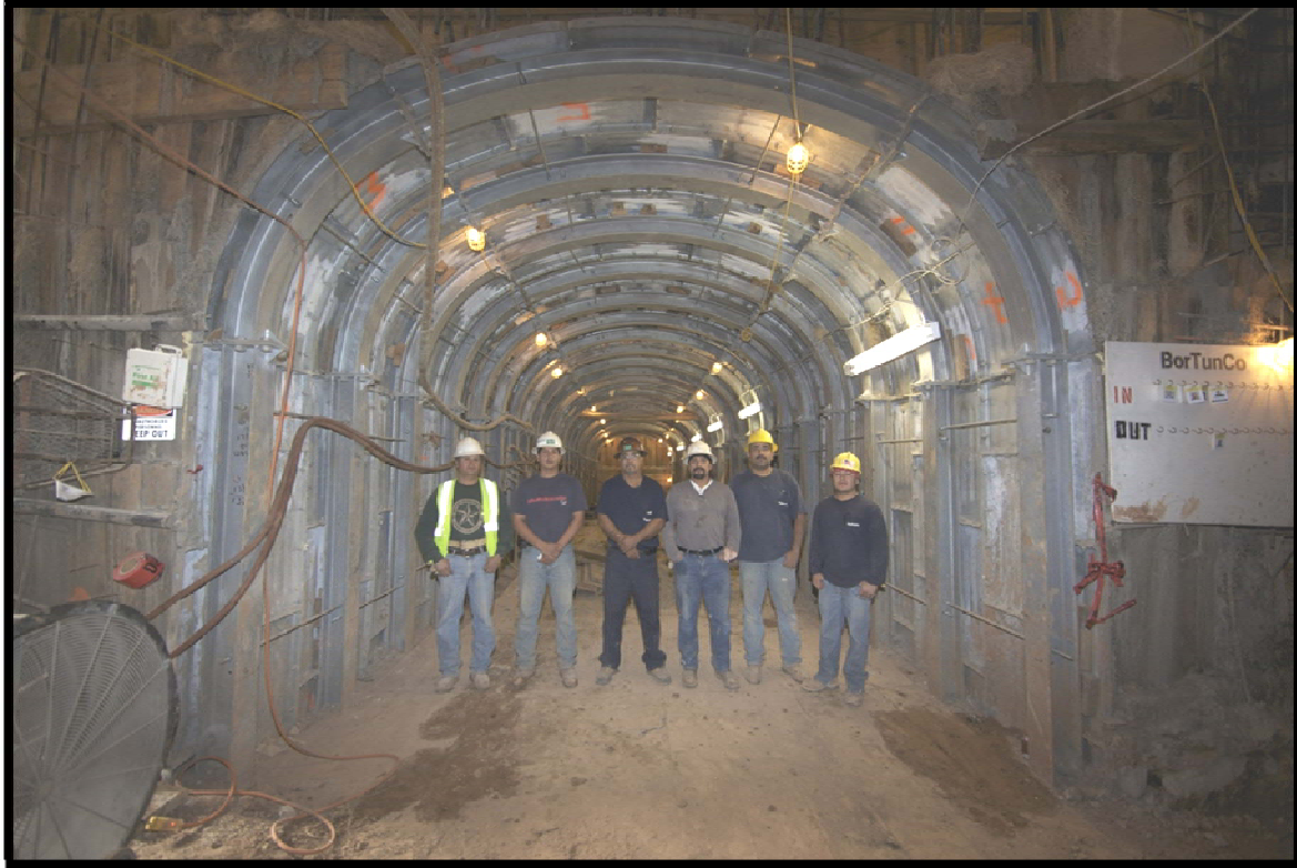
Completed 13.5' x 14.5' Arch Tunnel under (2) METRO Rail Lines
